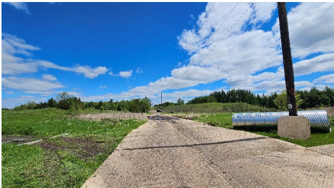
Powerline Corridor facing south from eastern edge of property – Xcel matting in place for pole replacement
