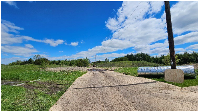
Powerline Corridor facing south from eastern edge of property – Xcel matting in place for pole replacement
