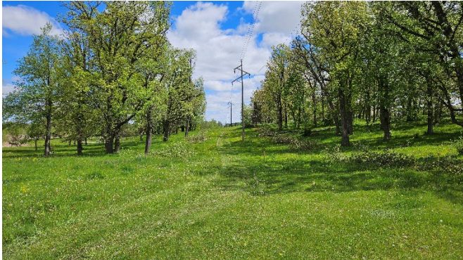
Powerline Corridor facing north from southern property line
