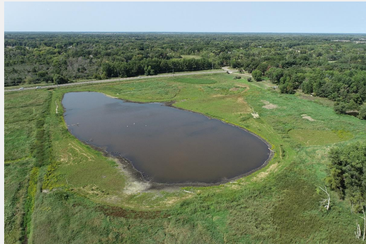
Aerial image of excavated wetland habitat
