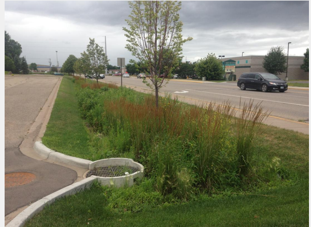
Stormwater “tree trenches”
