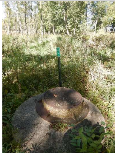
City of FL sewer manhole
