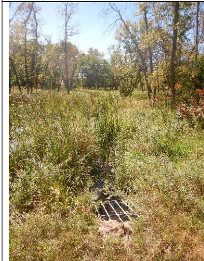
Culvert under North Shore Trail – flow from Cranberry Lake
