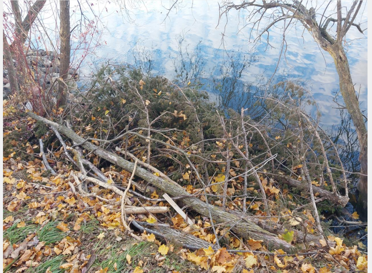
Cedar revetment installed on Bone Lake in November 2025
