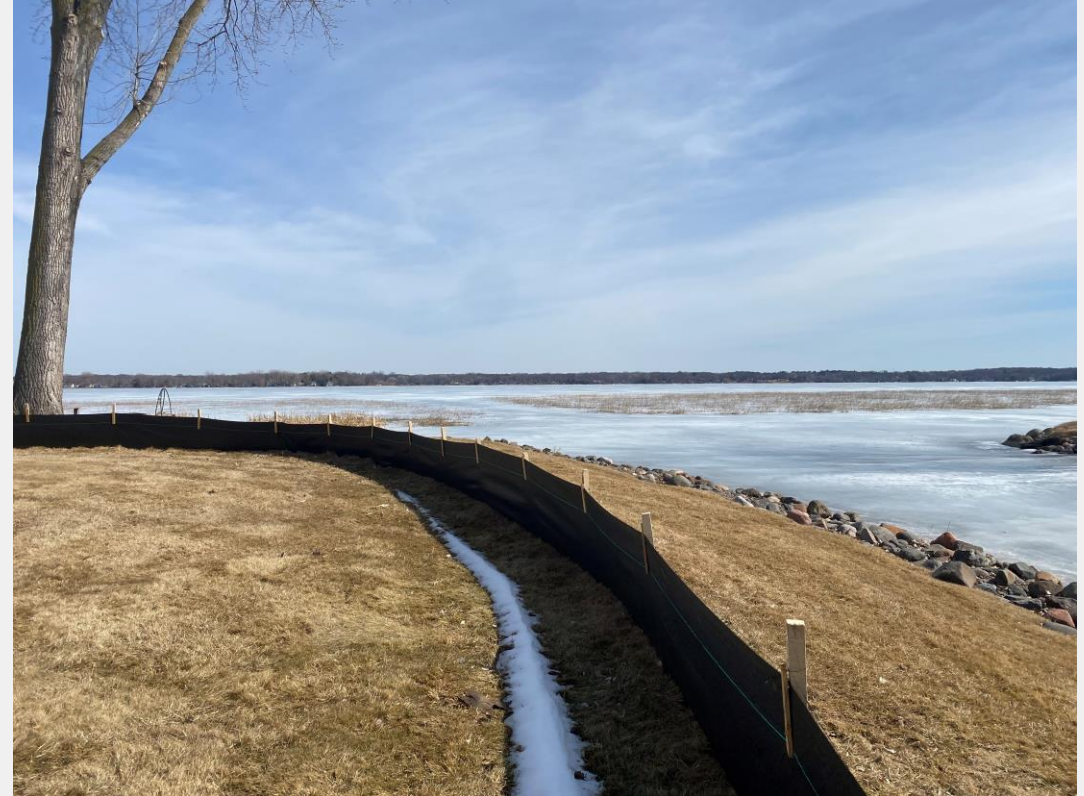
Silt fence installed at remodel site on Forest Lake's east basin
