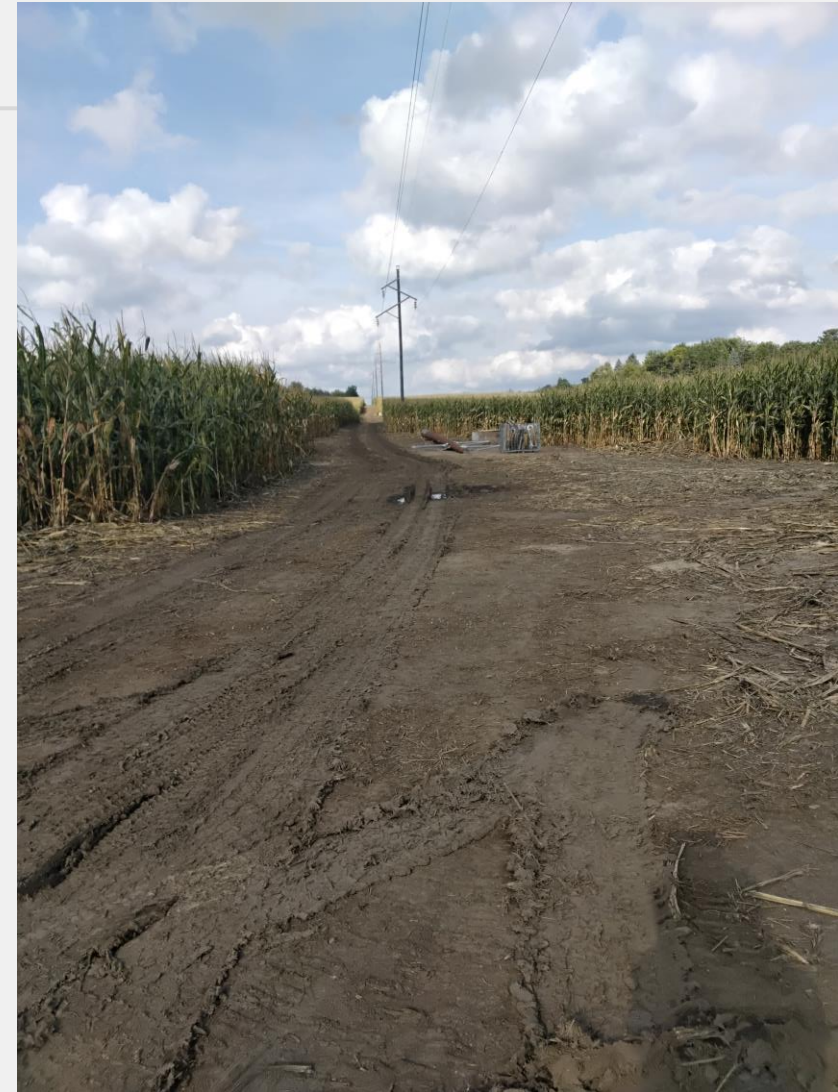
Xcel pole replacement project
