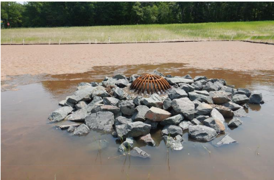
Filter bed inlet – water actively flowing into the filter bed.
