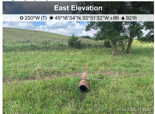
Photo 16: Center of subject property, north end facing west, culvert through field road
