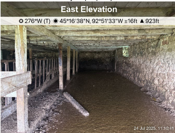
Photo 3: North end/former farmstead area interior view of barn
