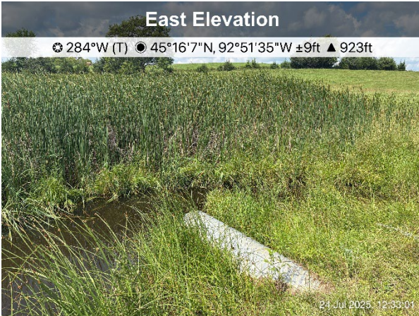
Photo 25: Center of subject property facing west, culvert through field road
