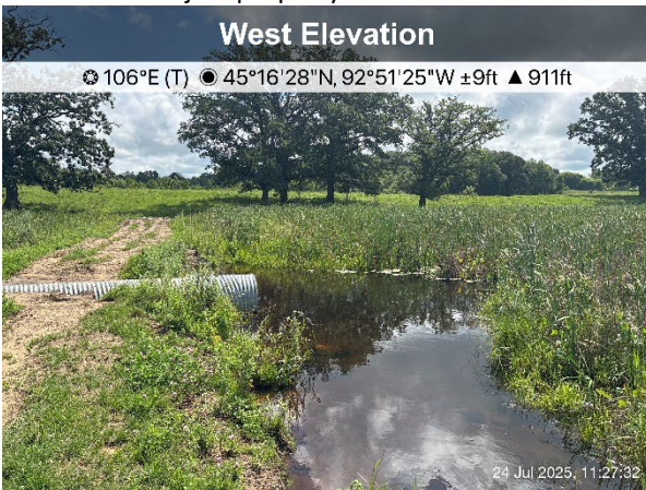
Photo 9: Center of subject property, north end, facing west, culvert through field road and wetland area
