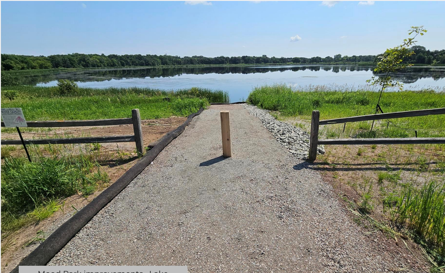
Mood Park improvements. Lake access repair completed.
