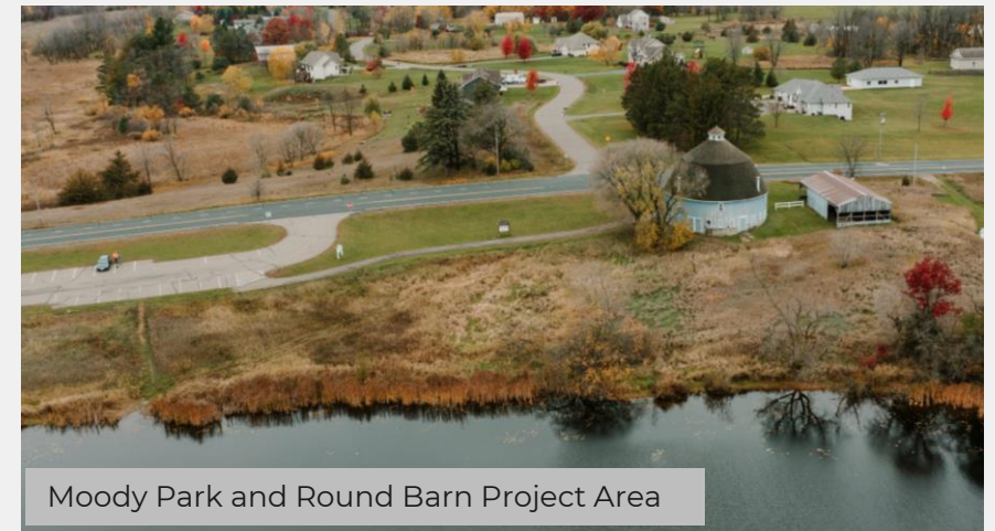
Legacy Load Removal Area
