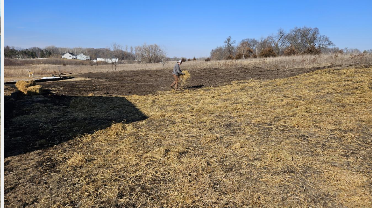
Spoils removed from area near Bone Lake. Site restored and stabilized.
