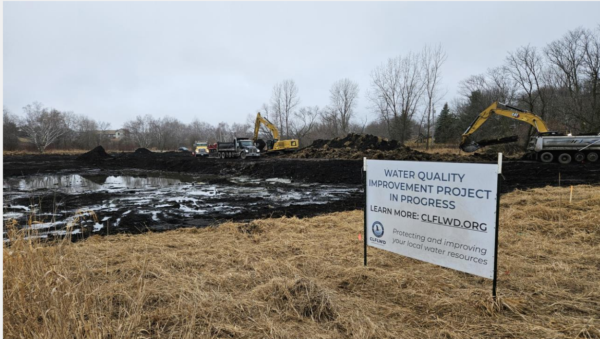
WJD6 Wetland Project Area. Excavation and haul.
