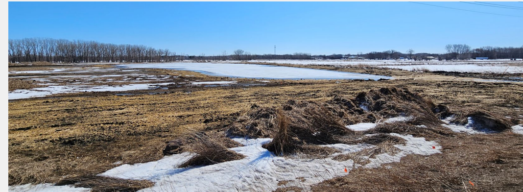
Excavated wetland filling with spring melt 03-28-23
