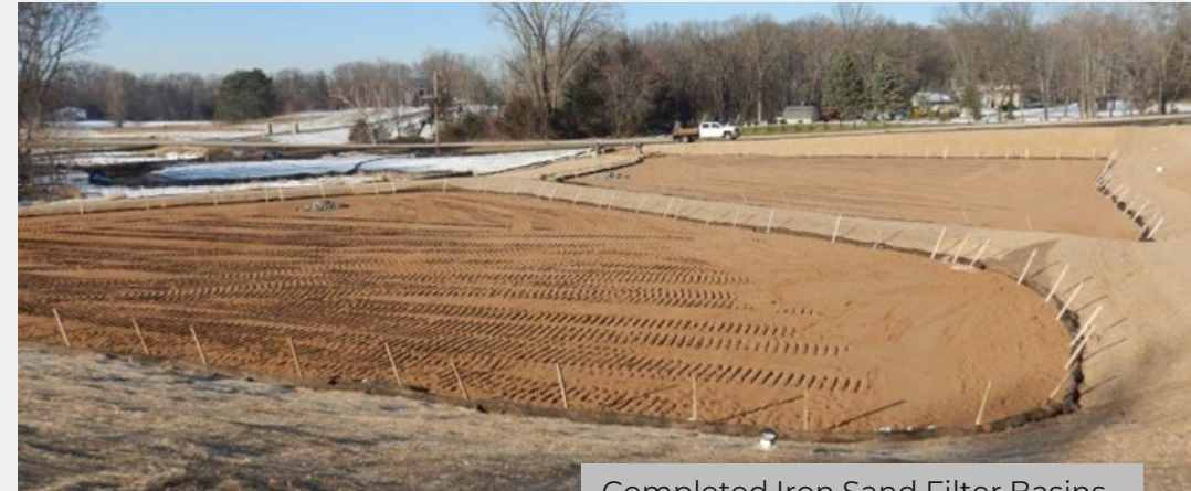
Completed Iron Sand Filter Basins
