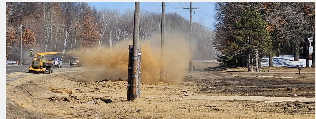
Site Restoration mulching in progress, 03-28-23.
