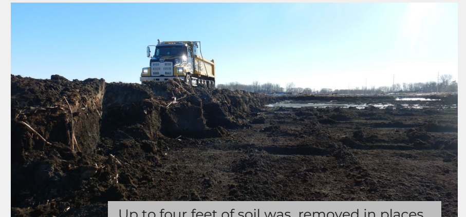
Up to four feet of soil was removed in places.
