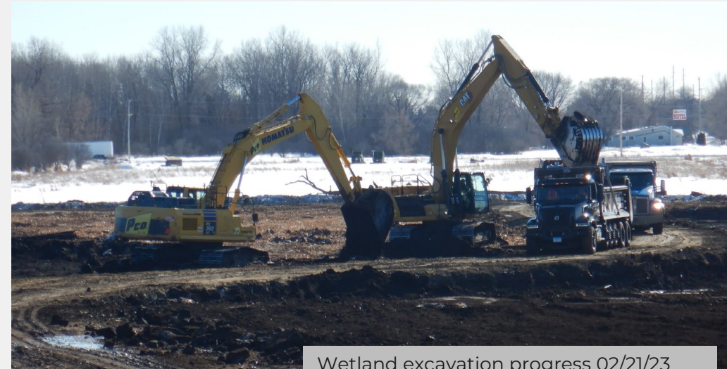
Wetland excavation progress 02/21/23
