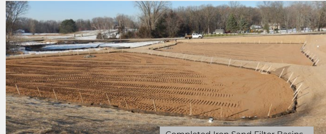
Completed Iron Sand Filter Basins
