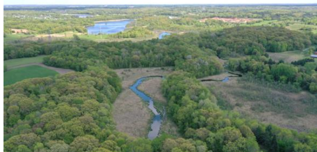
Aerial photo of School Lake outlet channel
