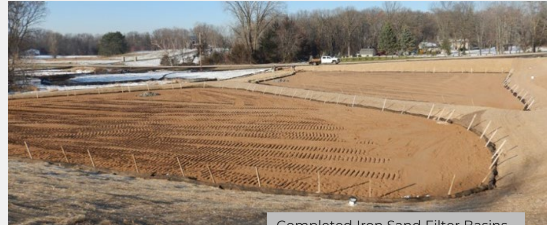
Completed Iron Sand Filter Basins
