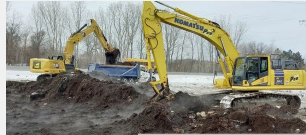
Wetland excavation progress 1/31/23
