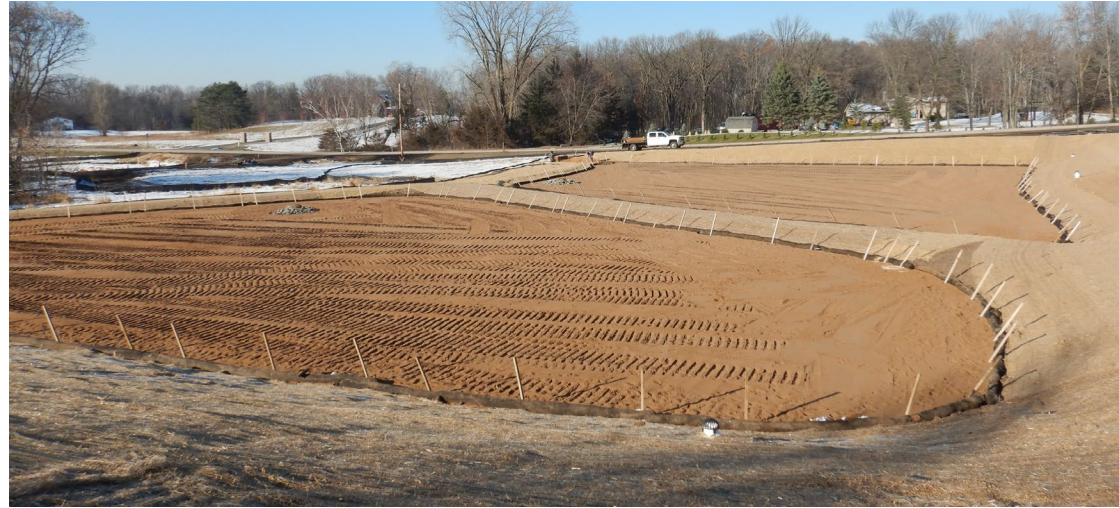
Completed Iron Sand Filter Basins.
