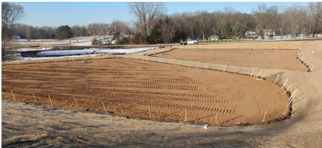
Completed Iron Sand Filter Basins.
