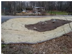
2012 – North Shore Trial & Hayward Ave. stormwater retrofit
