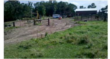
Feedlot Runoff Control project under construction – 2011 Program Project
