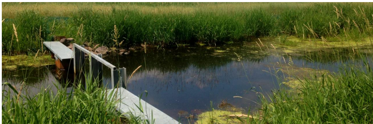
Manually operated weir at Bixby Park.
