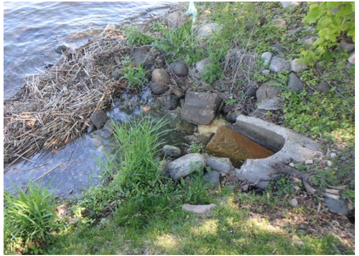
Existing outlet pipe to Forest Lake (5/17/16)
