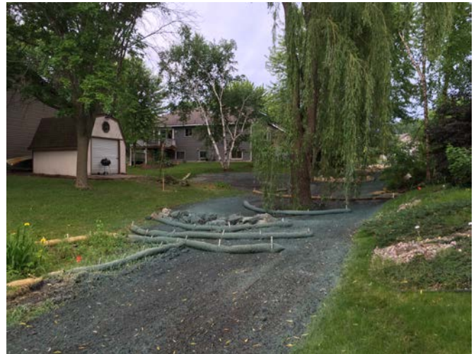
Channel stabilization in progress with erosion control (6/10/16)
