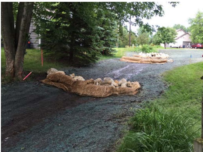
Rock check dams shortly after installation (6/10/16)
